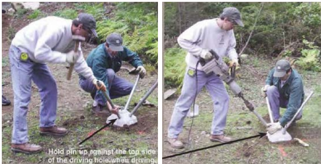
Photo 15.5 - Driving in a Diamond Pier Pin
