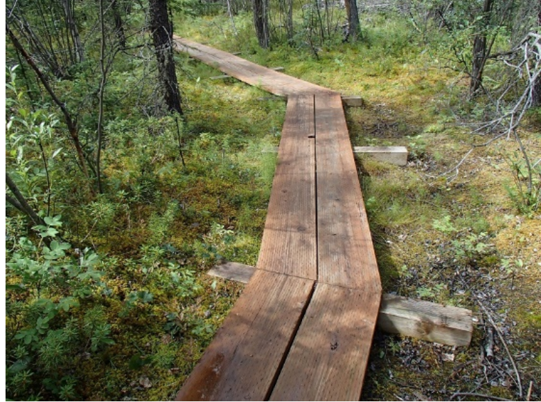
Photo 15.1 - Timber Planking Structure (left) and Curved Planking (right)
